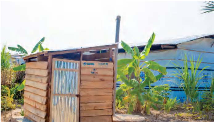
Photo of a semi-durable latrine constructed at the Mutambara internally displaced persons site in Rumonge.
