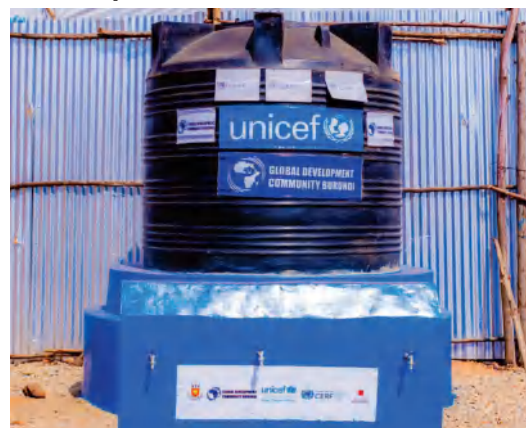
Drinking-water point with three taps constructed on the grounds of the Mubimbi health post with UNICEF support.
