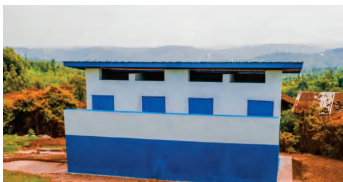
Image taken during the inauguration of WASH facilities completed in 10 health facilities in Kayanza, Kirundo and Musinga with UNICEF Burundi support
